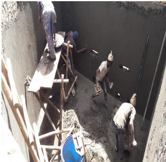
Plastering in process.
