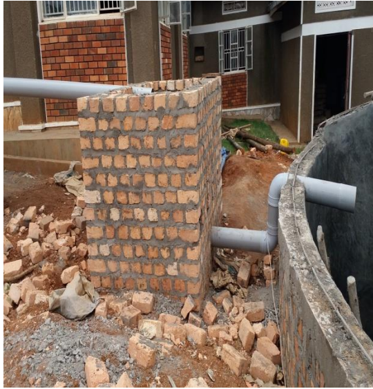
Connection from the filter to tank.
