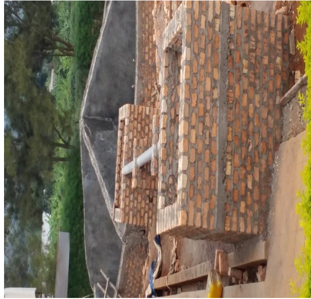
One Munhall to collect water and the filter.
